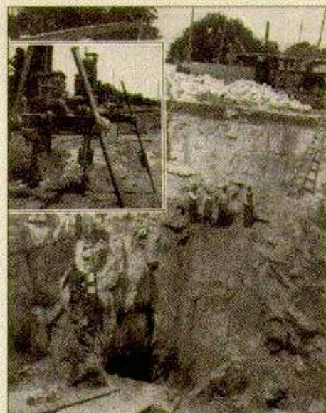
Fig. 11.—Rock Excavation for Counterweight Pit. Inset Shows Drills on Quarry Shaft.
