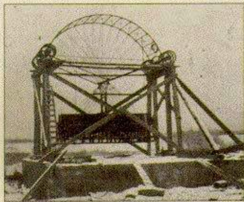
Fig. 7.—Car Erected on Roof of Thompson's Point Station, Ready for Test.
